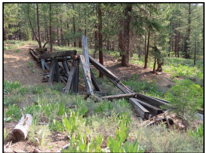
Remains of a trestle for a long-abandoned logging railroad
